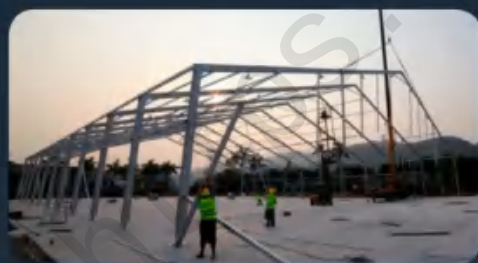
Trial Installation before Loading
