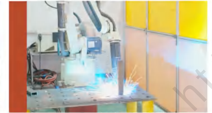
Robot welding operation
