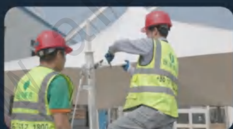
Trial Installation before Loading
